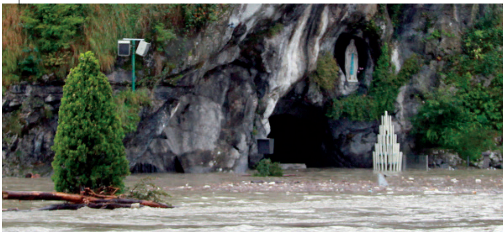
Flooding at the Grotto, Lourdes
